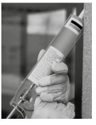
when one-part silicone construction sealants entered the marketplace. One of the first single-component silicone sealants was a clear acetoxy sealant from Dow Corning. In 1958, that sealant was used as a weatherseal in a building on the western shore of Lake Michigan.
